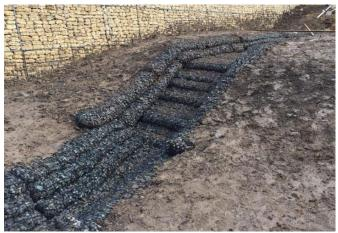
The cascading channel lined with the Rock Rolls and Rock Mattresses are delivered to site ready filled, lifted off the lorry and lowered into place on the prepared graded profile.
